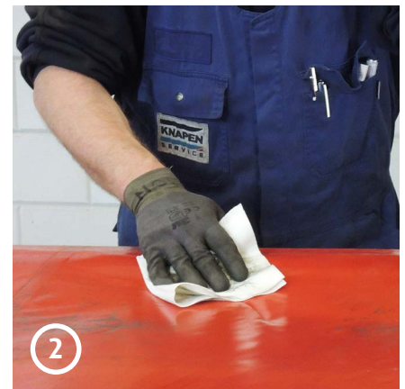
2 Make sure that all dirt, grease, oil, etc. is removed from the surface to be repaired. Ensure that the surface is completely dry before applying the tape
